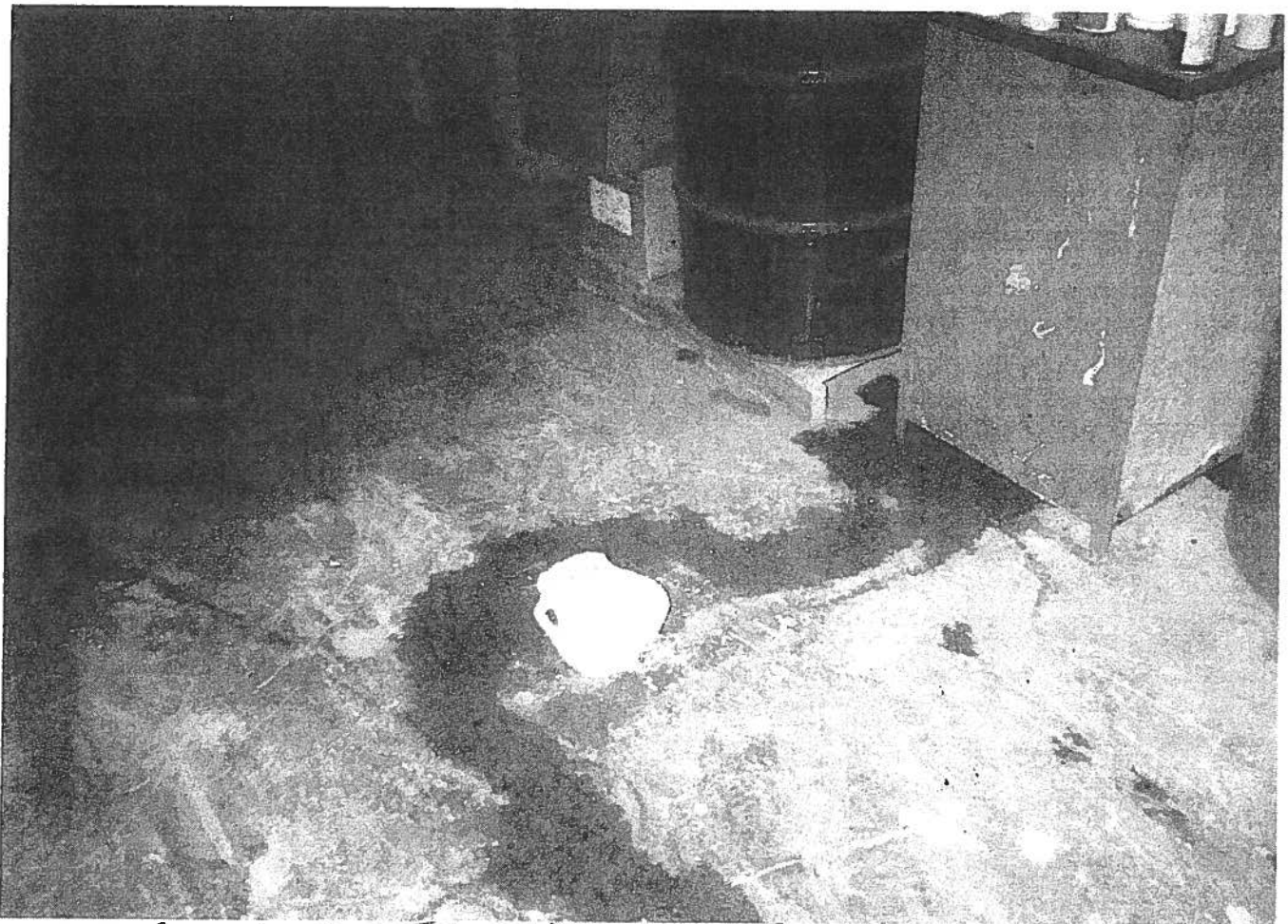
1ST FLOOR, NORTH SIDE - RED FLAMMABLE STORAGE
