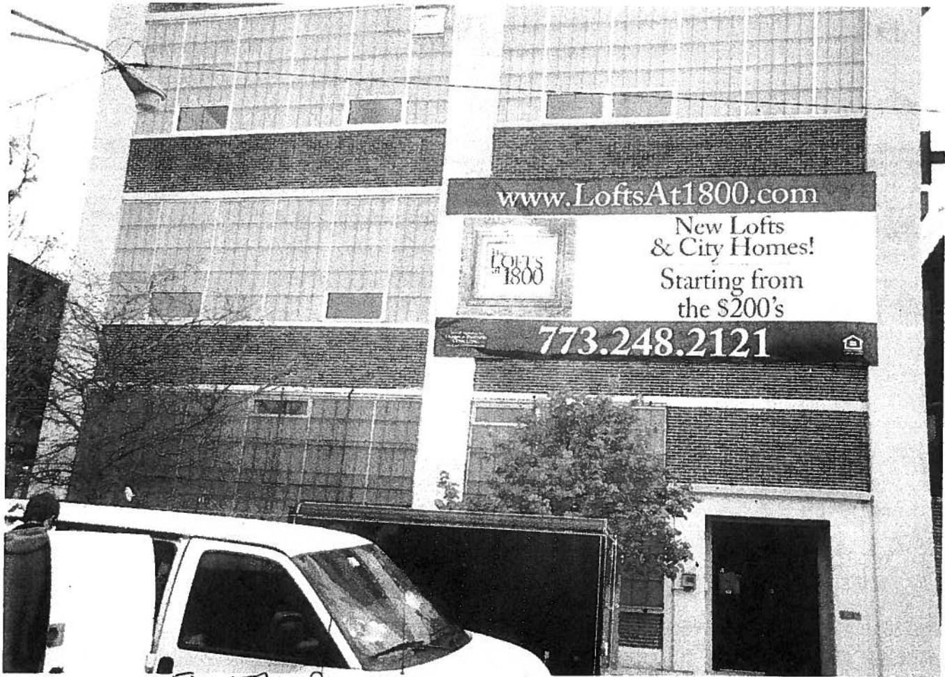
EXTERIOR, 1810 W. GRACE ST
